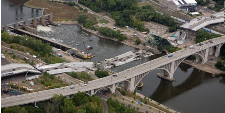
Figure 2-5: I-35W Bridge collapsed, Minnesota, USA.
