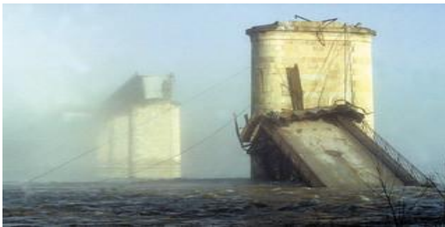
Figure 2-6: Hintze Ribeiro Bridge disaster, Portugal.
