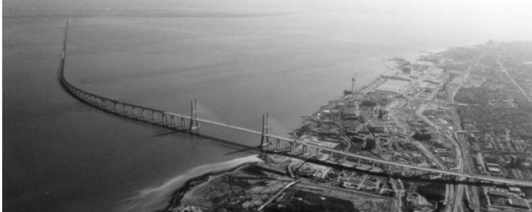
Figure 2-8: Ponte Vasco da Gama, Lisbon, Portugal.
