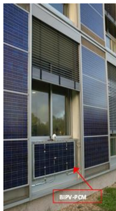
Fig. 1, Prototype installed on the SolarXXI main façade
