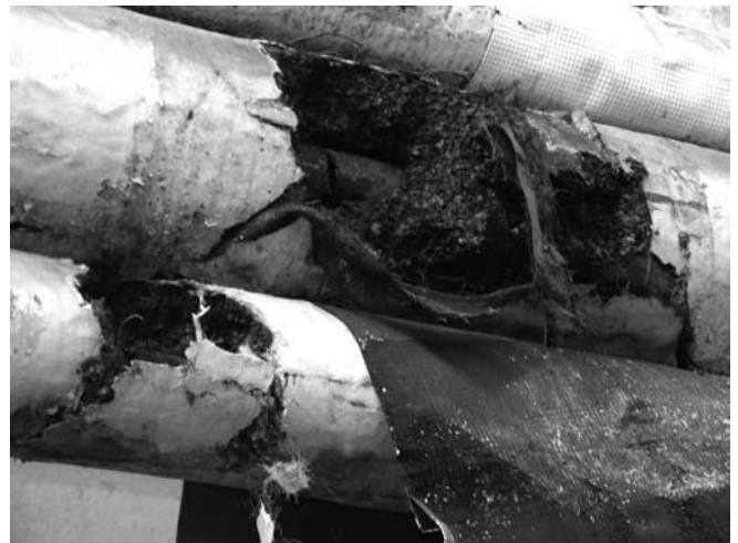
Fig. 4. Cooling pipes with ICB insulation before demolition.
