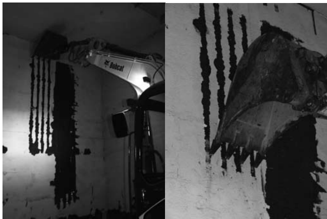
Fig. 6. Operation for the removal of ICB from the cold chambers walls.
