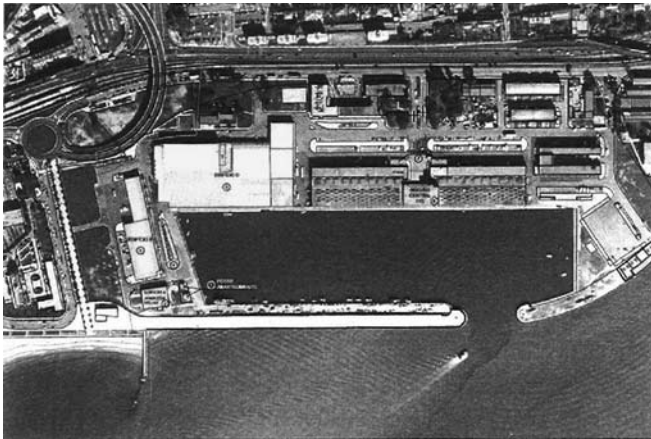
Fig. 1. Aerial view of the demolition site with buildings for demolition in white (left corner of the dock).
