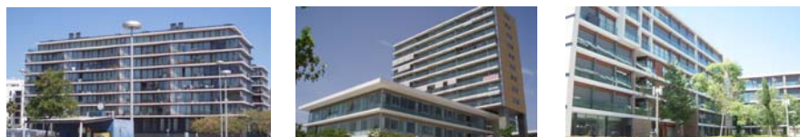
Fig. 3. Residential buildings with glass façades (Lisbon, last years).
