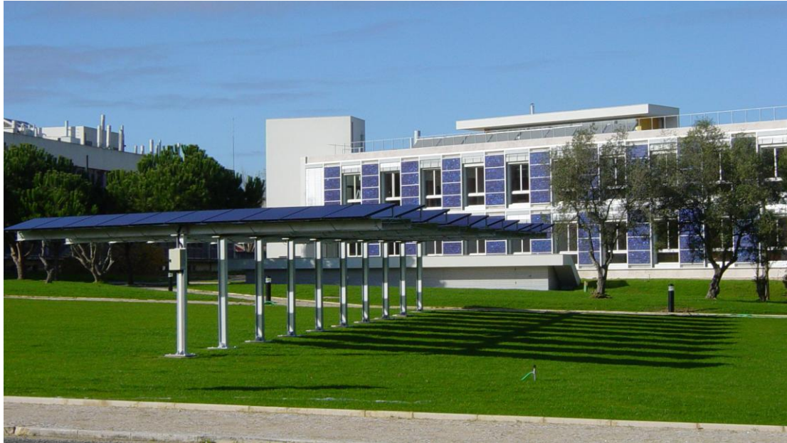
Fig. 1. The Solar XXI Building and the PV systems installed, in the façade and in the car park area.
