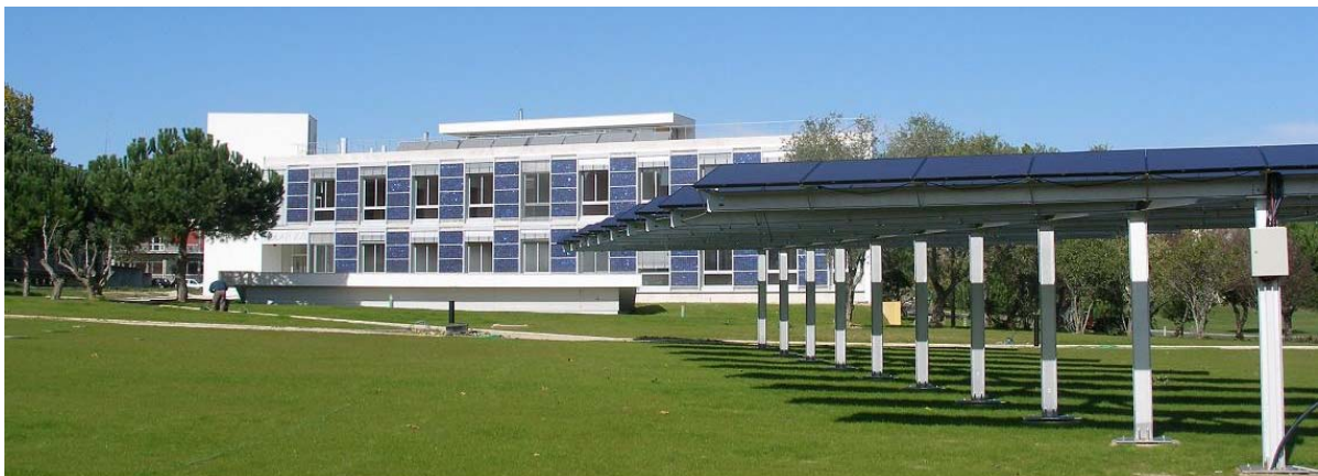
Fig. 12.The Solar XXI Building and the PV system in the car parking.
