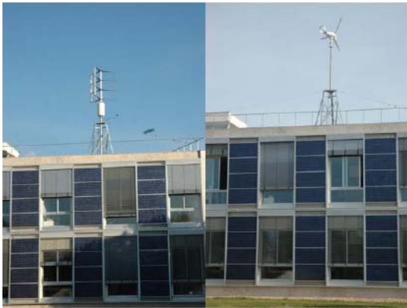
Fig 4. Passive Solar Building XXI with small wind prototypes (test)
