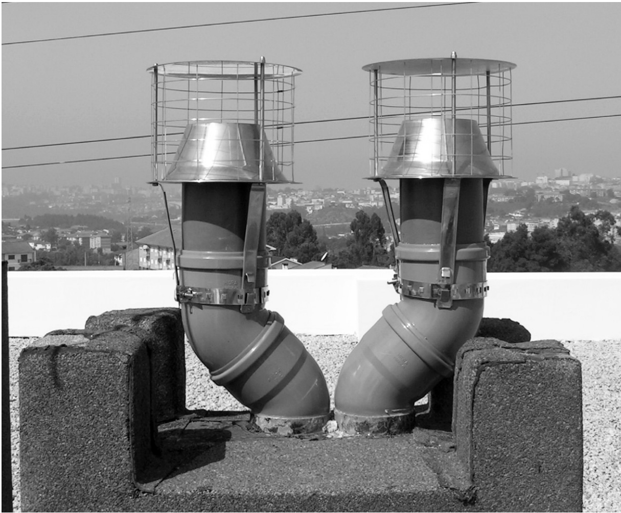
Fig. 4. Static ventilators on the bathroom ducts.
