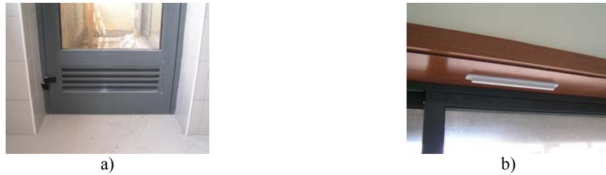
Figure 4: Air intake devices, a) fixed inlets for air intake in the kitchen, b) self-adjustable inlets for the air intake in rooms and living room
