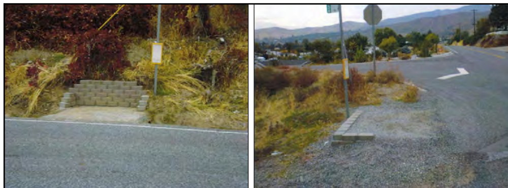
Figure 39. Rural Bus Stops Improved Using "Rhino Snot"
