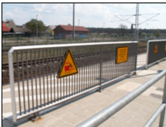
Figure 11. Barriers at Hamburg, Germany Platforms
