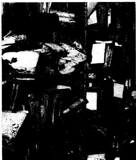
Fire Damaged Stacks. One Day after the Fire.
