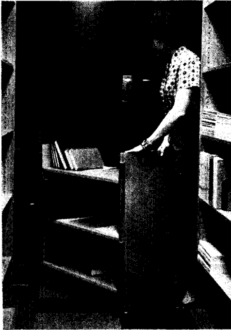
The small elevator connecting the stack areas is just large enough to carry a loaded book truck.
