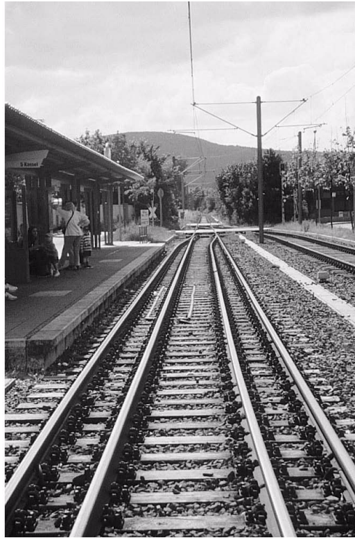
Figure 7 Example of Gauntlet Tracks
