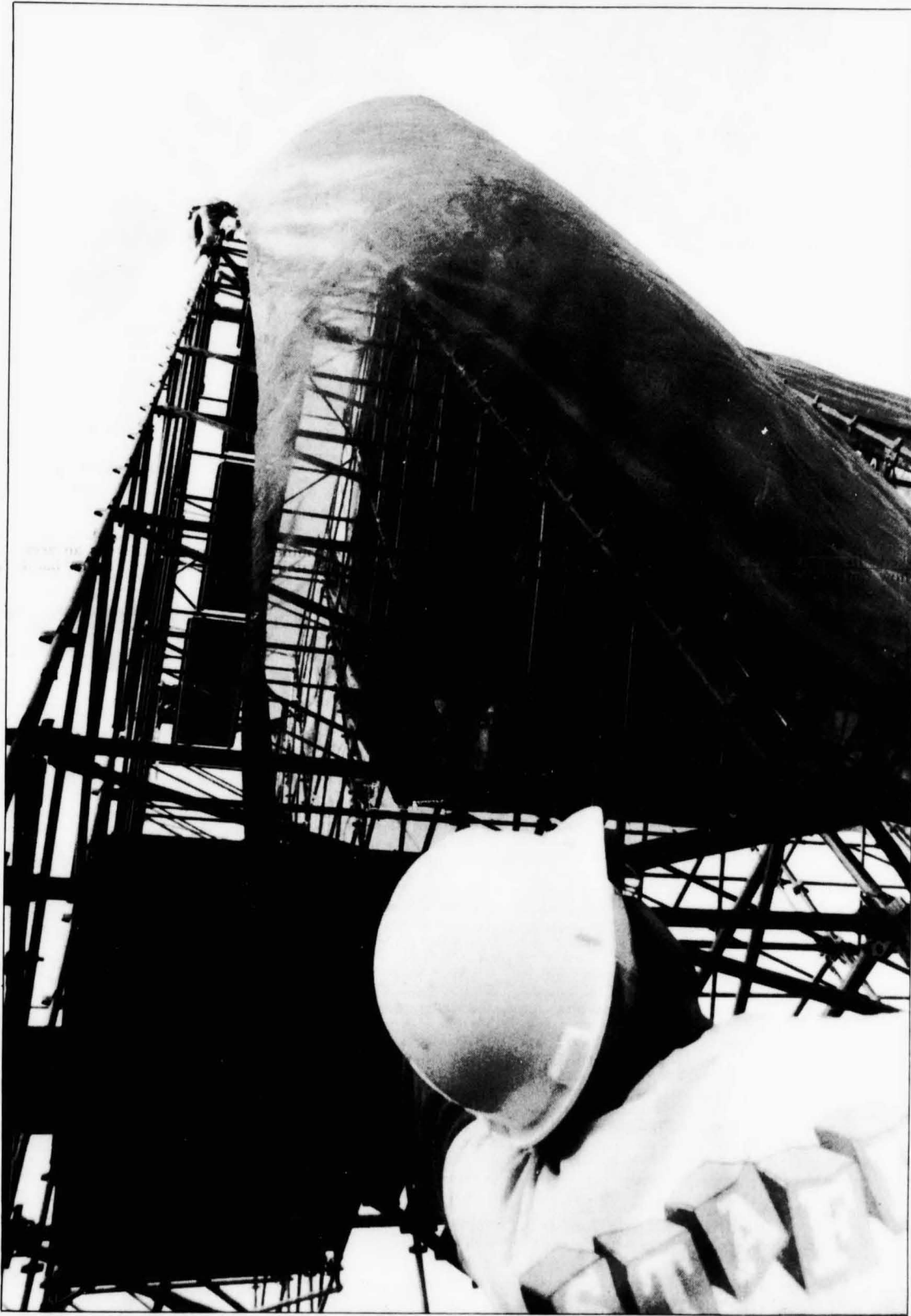
ABOVE: Stagehand Roger Clark keeps an eye on the direction of the wind skirt being put in place before the Pearl Jam concert at Spartan Stadium. The 16-by-40-foot skirts protect the performers and equipment from wind and bad weather.
