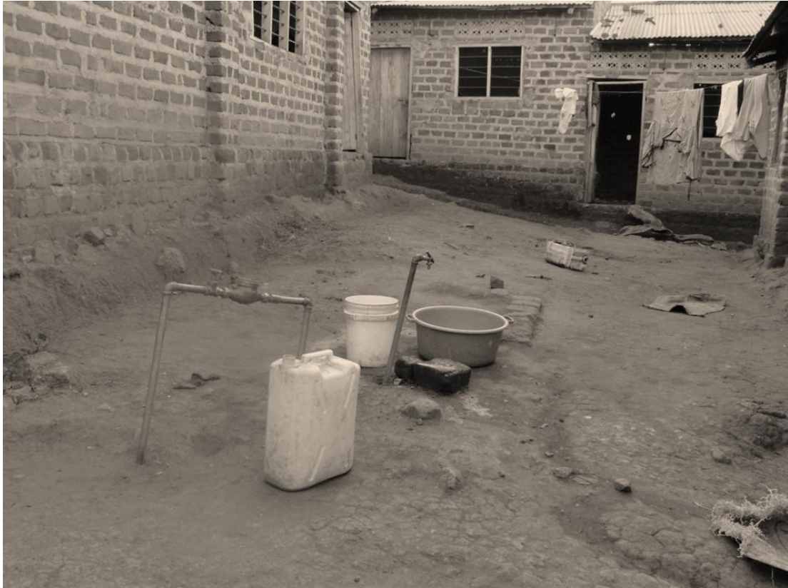
Figure 19. Mpigi Town metered yard connection.
