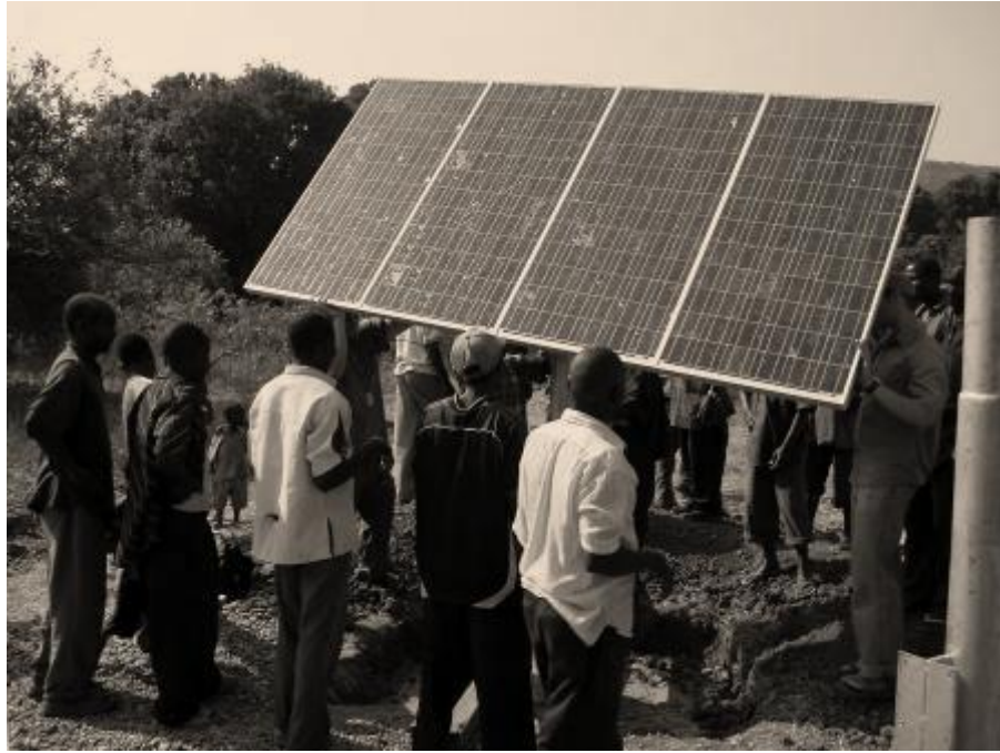
Figure 17. Installation of the solar array.
