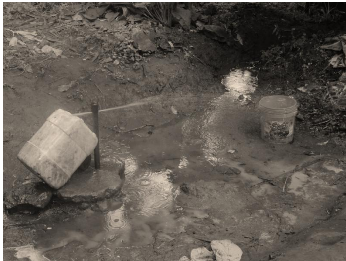
Figure 23. Illegal water source in a mountain community of Tanzania. A pipe planted in the gravity water distribution line traversing a village without appropriate water supply en route toward a village downhill.
