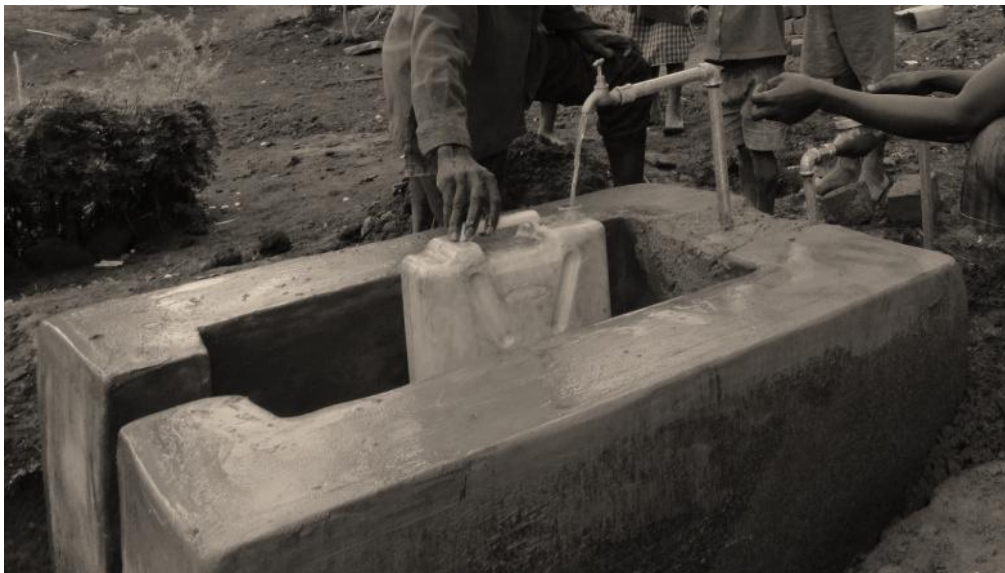
Figure 20. A completed tap stand in Kizzi.
