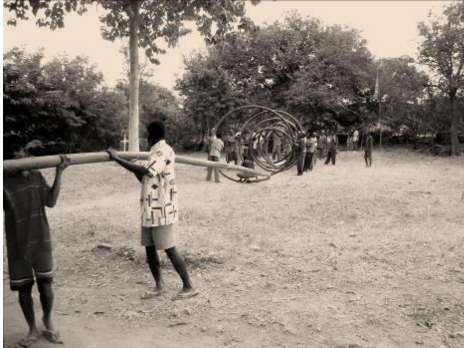
Figure 15. Laying PE pipes in Ngelenge.
