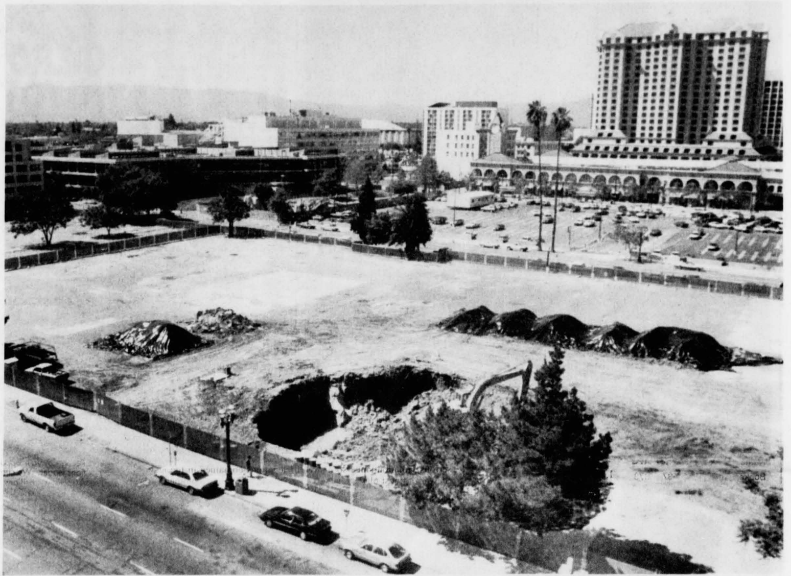
Piles of contaminated soil in photo above surround hole from which gas and oil tanks were removed. Fourth Street runs from lower left to lower right.
