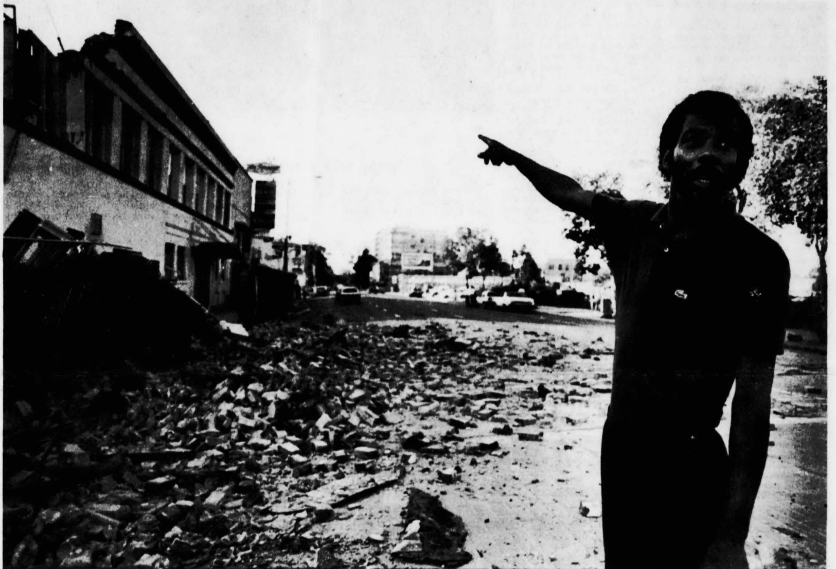
Calvin Miles points out the collapsed east wall of the gutted Marquis Apartment building
