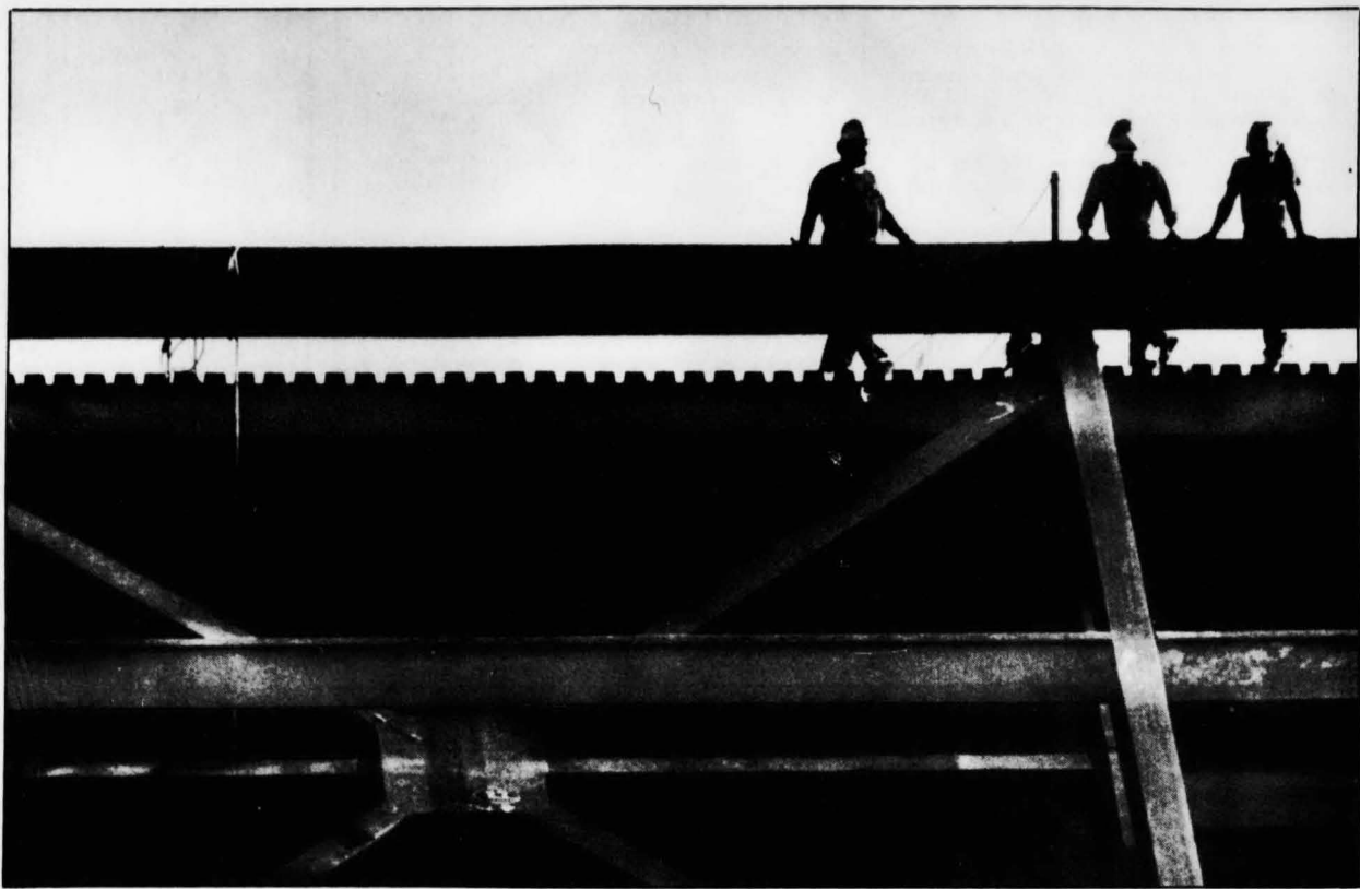
Brian Baer — Special to the Daily Three construction workers stand atop of the Student Union Recreation and Events Center. The project, which costs more than $20 million, was originally scheduled to open in September 1988 but may now open in July 1989 because of proposed structural changes.
