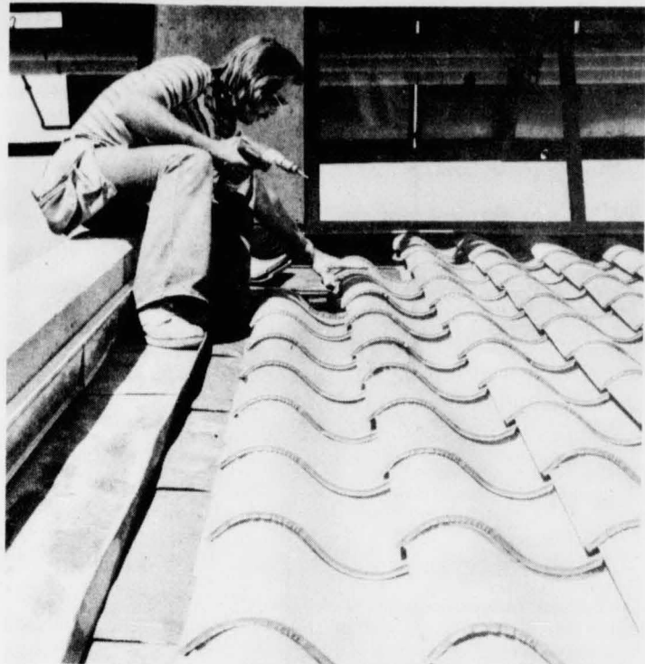
A construction worker lays down tile with aid of a power drill on the south entrance of the new Robert Clark Library.
