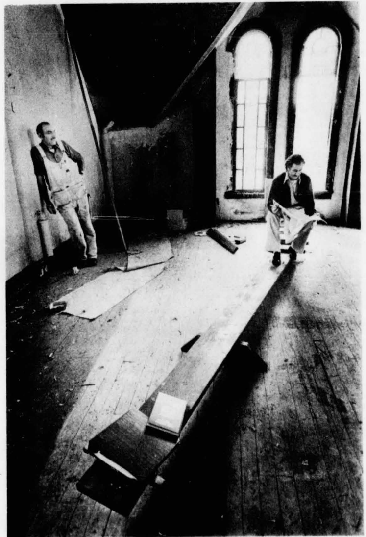
Carpenters Tony Serrano (left) and John Paride stand by for installation of chair.
