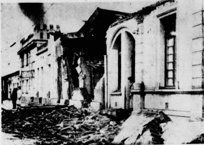
RUIN AT CONCEPCION —Standing between two old buildings, a relatively new structure was completely destroyed by severe earthquakes at Concepcion, Chile. Four new earthquakes hit southern Chile yesterday, bringing
