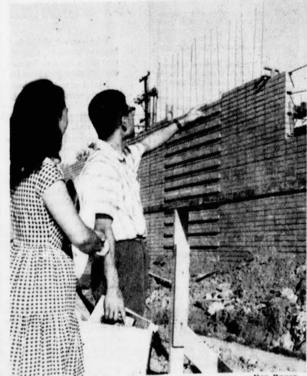
NEW FACES, NEW PLACES—Naoko "Nancy" Takaura and Ajo Yamasaki, Okayama, Japan students who are now attending San Jose State, stop to admire the new campus construction. The students were brought here through the Pacific Neighbors of San Jose and are living with families here.
