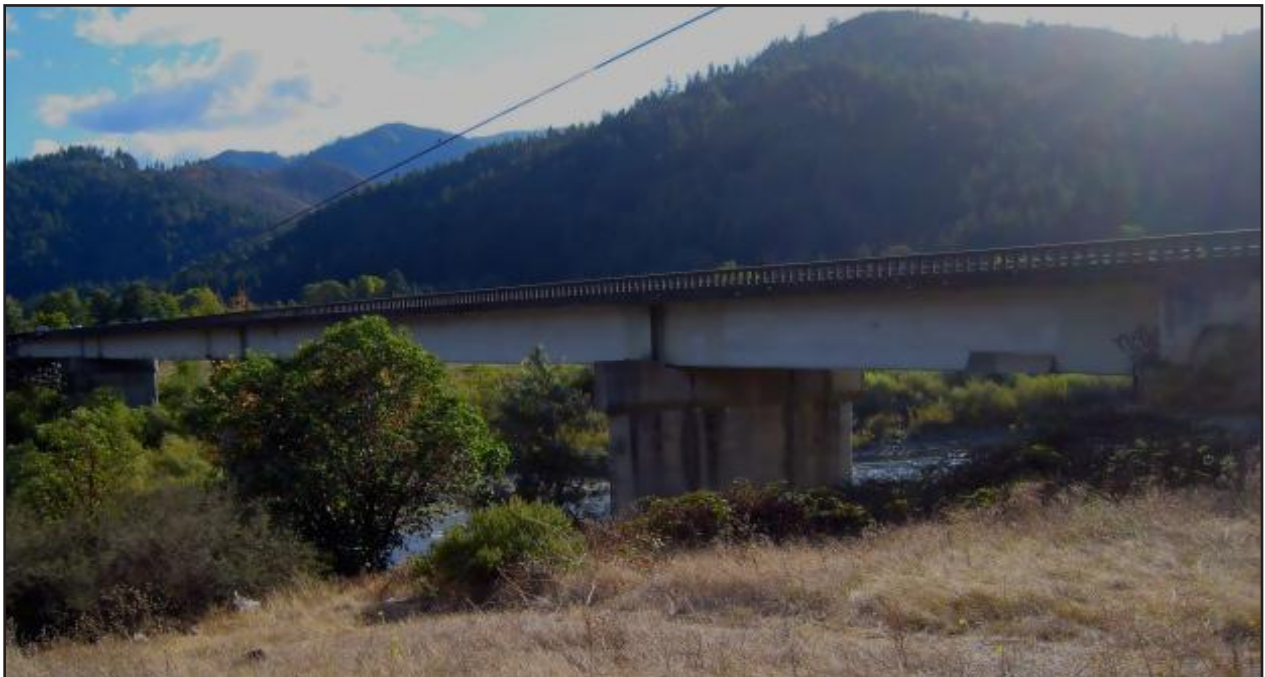
Figure 25. The Trinity River Bridge Underpass
