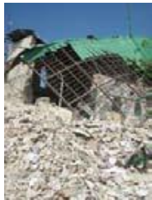
Haiti Earthquake: Ministry of Public Works
