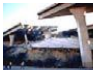
Highway vulnerability to Northridge Earthquake
