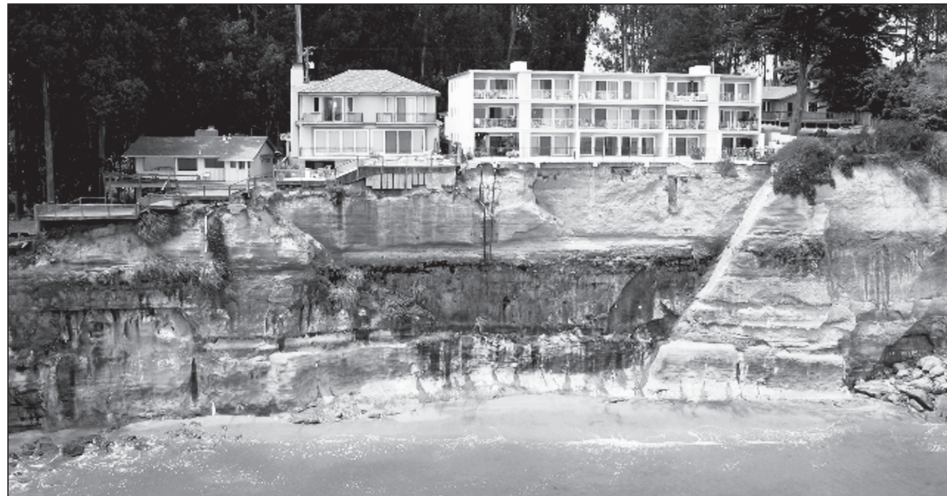
Ocean Beach succumbs to shoreline erosion from long-term rising sea levels and stronger winter storms. Photo courtesy of Gary Griggs / UCSC
