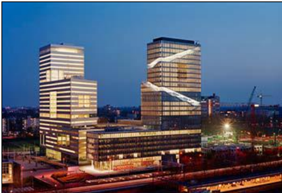
Figure 2. HSR Station in Zuidas district of Amsterdam
