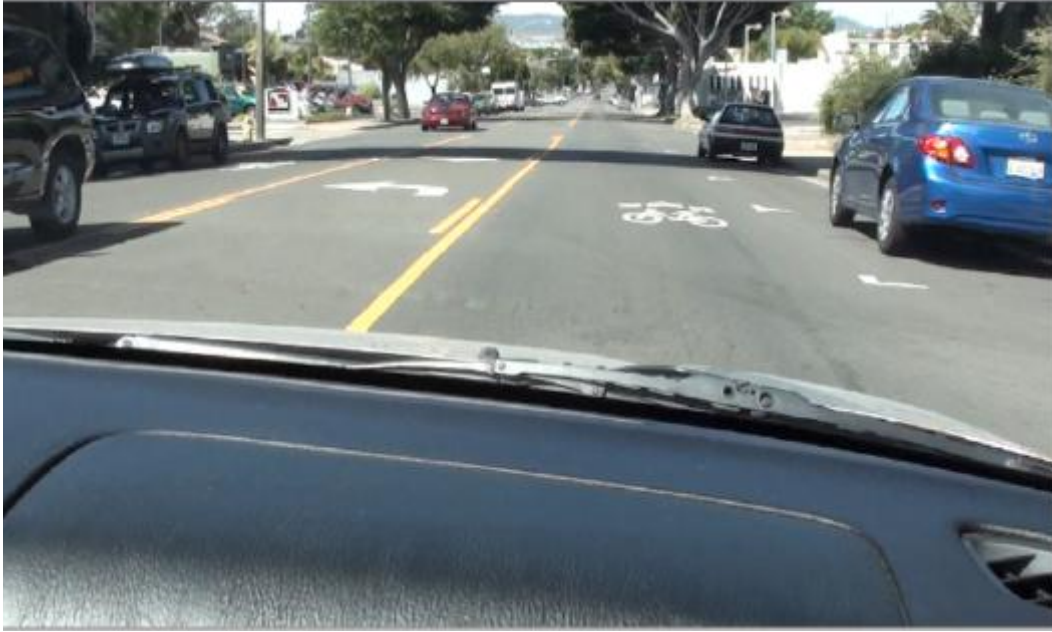
Figure 21. Shared Roadway (Sharrow) – San Luis Obispo, California
