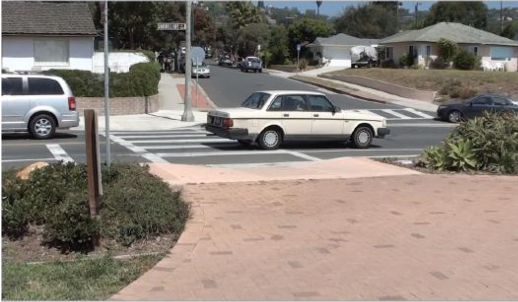
Figure 37. Narrowed Pavement at Intersection to Shorten Crossing – Santa Barbara, California
