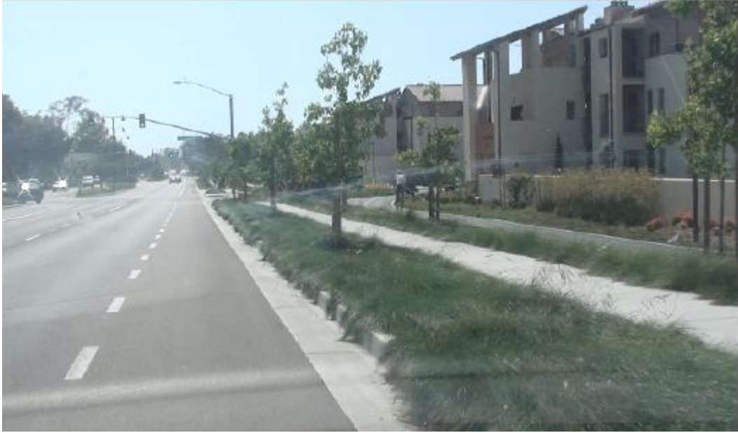
Figure 17. On-street Bicycle Lane with Parallel Side Path – Santa Barbara, California
