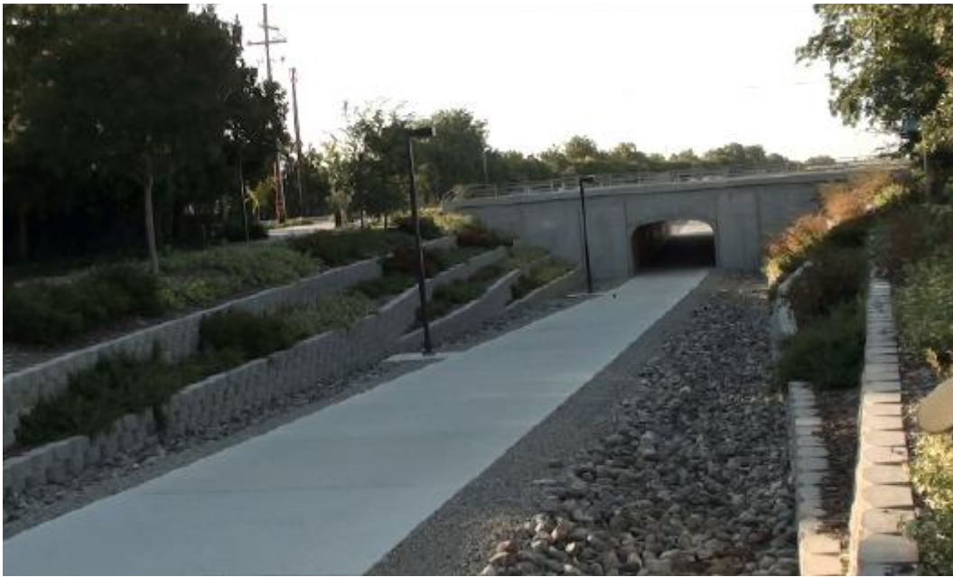
Figure 47. Underpass for Bicycle Path #2 – Davis, California
