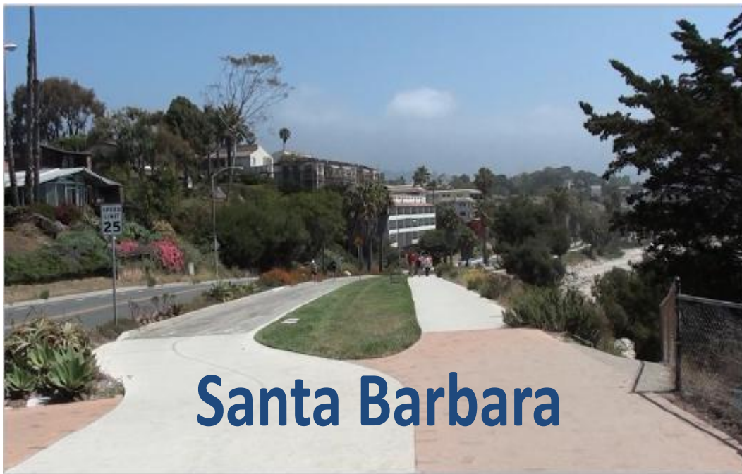
Figure 15. Separate Walking, Bicycling and Auto Facilities – Santa Barbara, California
