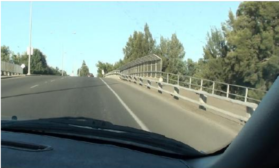
Figure 48. Bicycle Lane on Highway Bridge – Davis, California
