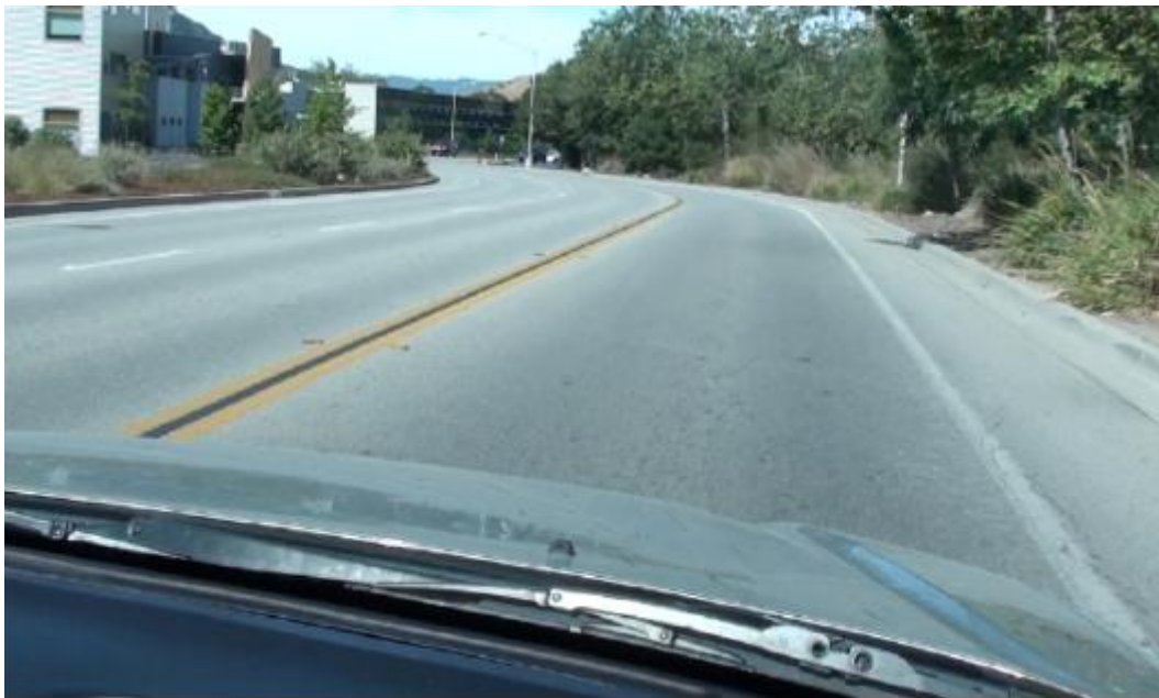
Figure 28. Wide Shoulder for Walking and Parking – San Luis Obispo, California
