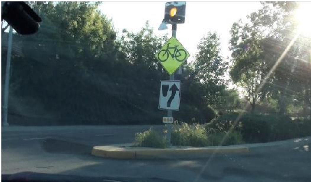
Figure 36. Bicycle Only Signal along Non-Motorized Route – Davis, California
