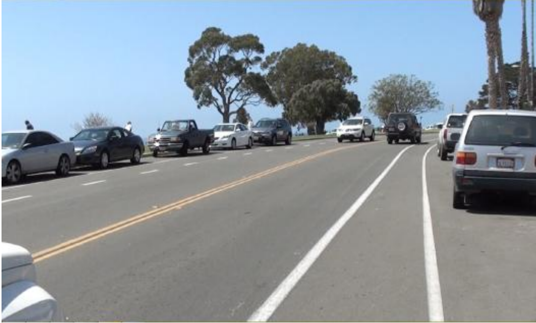
Figure 23. Divided Shoulder for Parking and Bicycling – Santa Barbara, California
