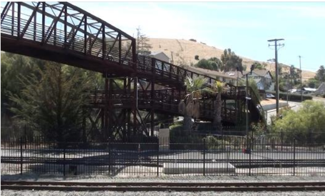
Figure 44. Pedestrian and Bicycle Overpass over Railway Line – San Luis Obispo, California
