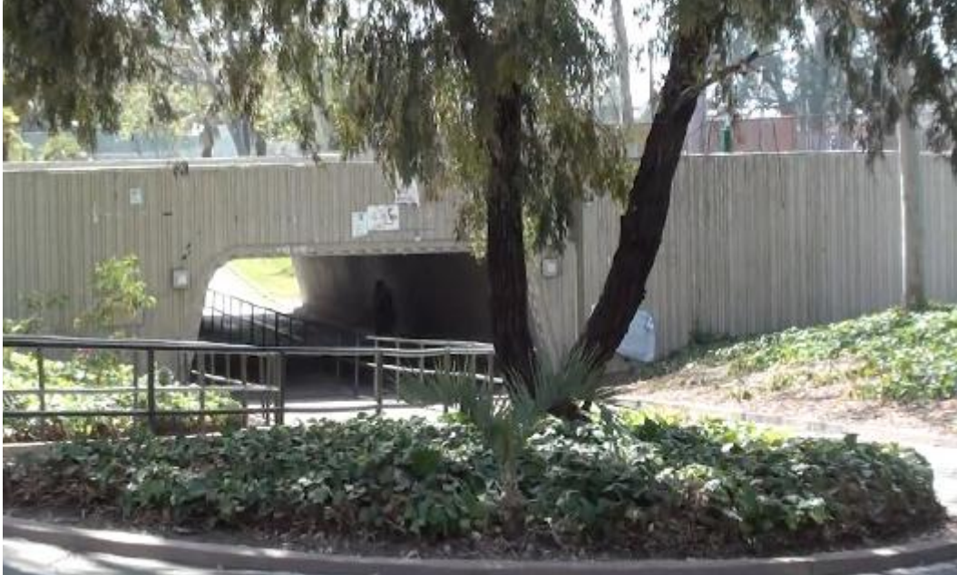
Figure 46. Underpass for Bicycle Path #1 – Santa Barbara, California
