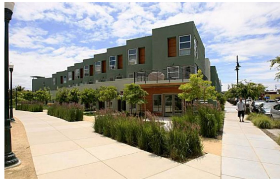
Figure 11 New Project Entrance to the Doyle Street Greenway
