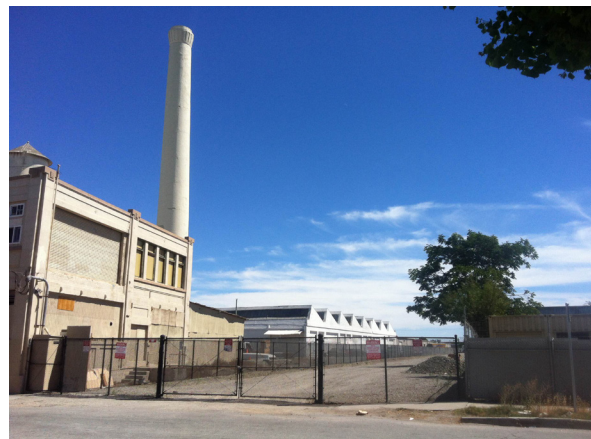
Figure 7 American Can Company and 4th Street Line, View from Martha Street
