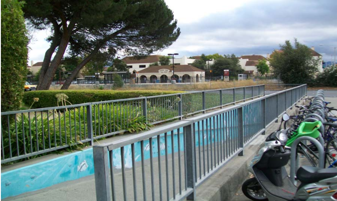
Figure 6: View of California Avenue Caltrain station with pedestrian tunnel entrance in foreground. Photograph by author.
