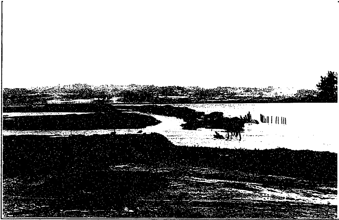
Figure 7.--Breached Levee at Moss Landing Wildlife Area
