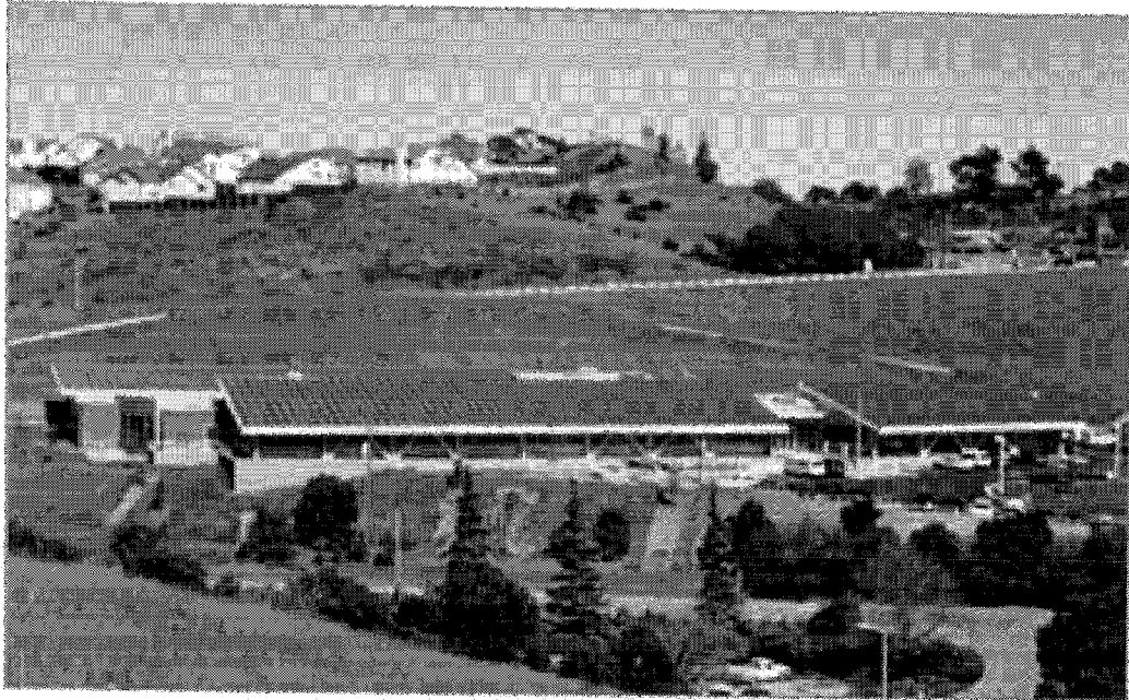
234 kW PV System on Forensics Lab in San Mateo, California
