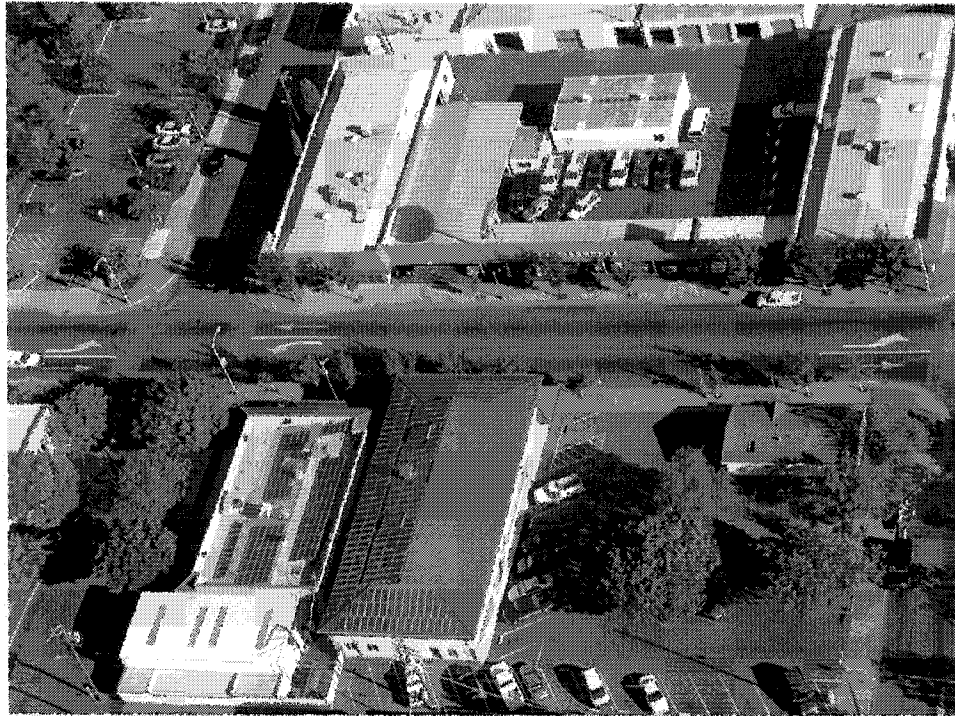
PV System in Oroville, California
