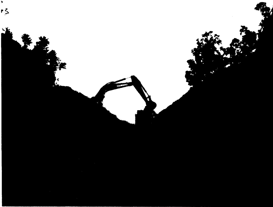
Figure 2.2. Road Construction Observed in Palau, March 2005
