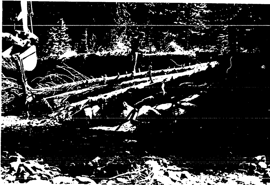
PHOTOGRAPH 11. Detailed View of Boulder-Log Structure
