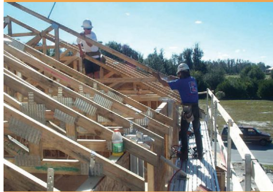
From top: Photo 3 shows the guardrail device in place at a construction site, while Photos 4 and 5 show the hanging scaffolding system in use (hanging exterior and interior to the structure).
