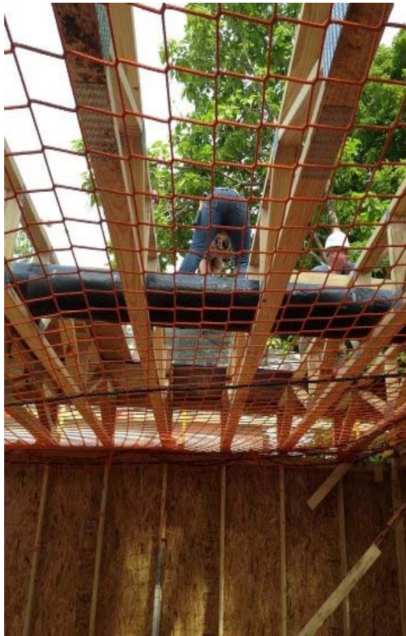
Figure 1 – Safety nets guard workers on second floor.
