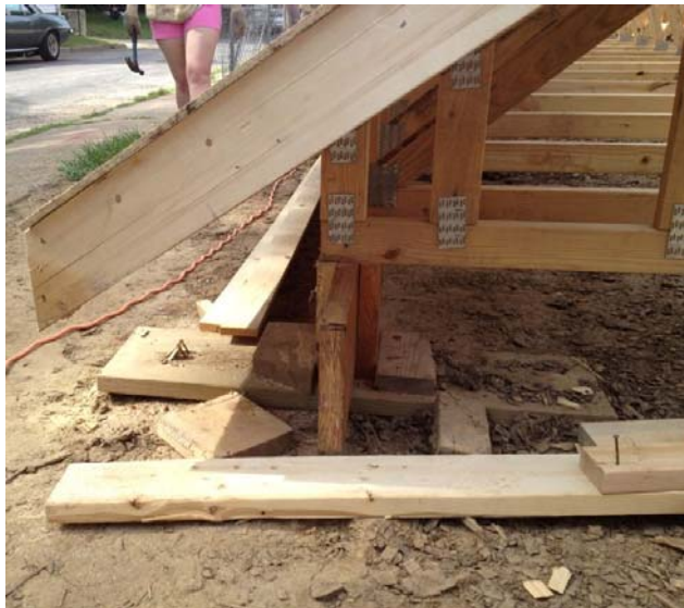
Figure 11 – Roof assembly built on stationary base.
