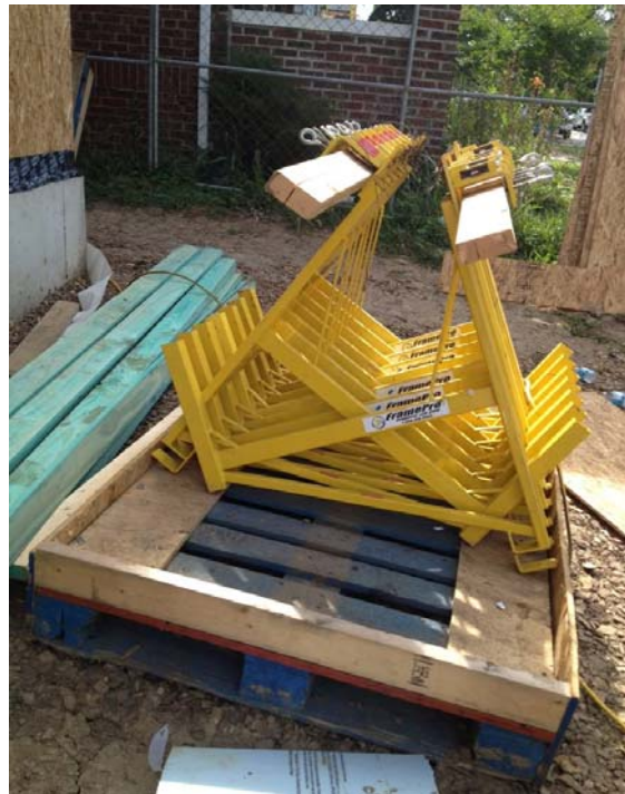
Figure 8 – Storage bin for hanging scaffold storage/transport.
