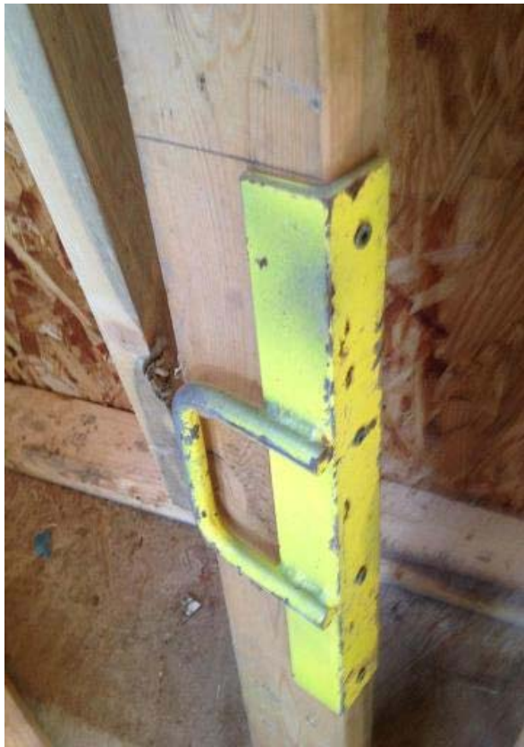
Figure 3 – Fabricated bracket for safety net.
