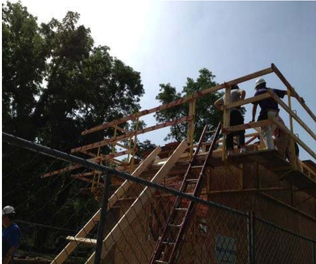
Figure 5 – Hanging scaffold system in place.
