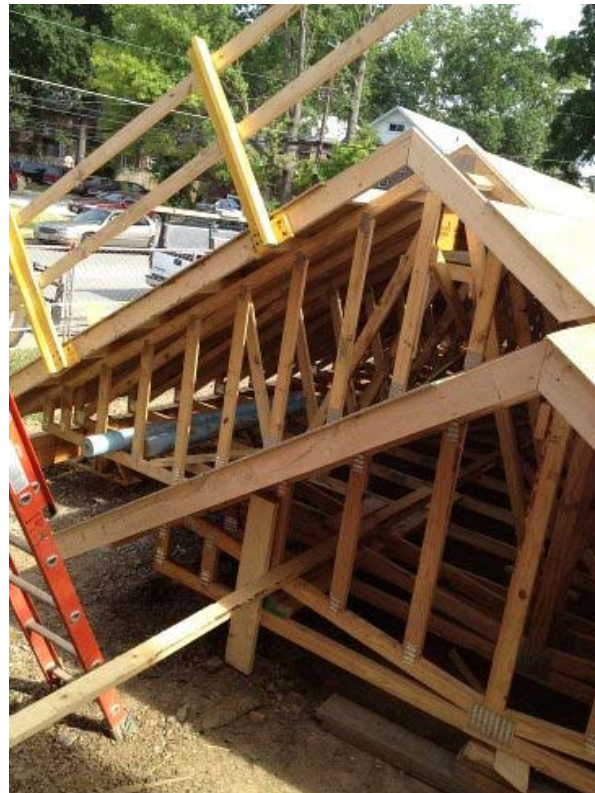
Figure 12 – Guardrail protects the gable end of truss.
