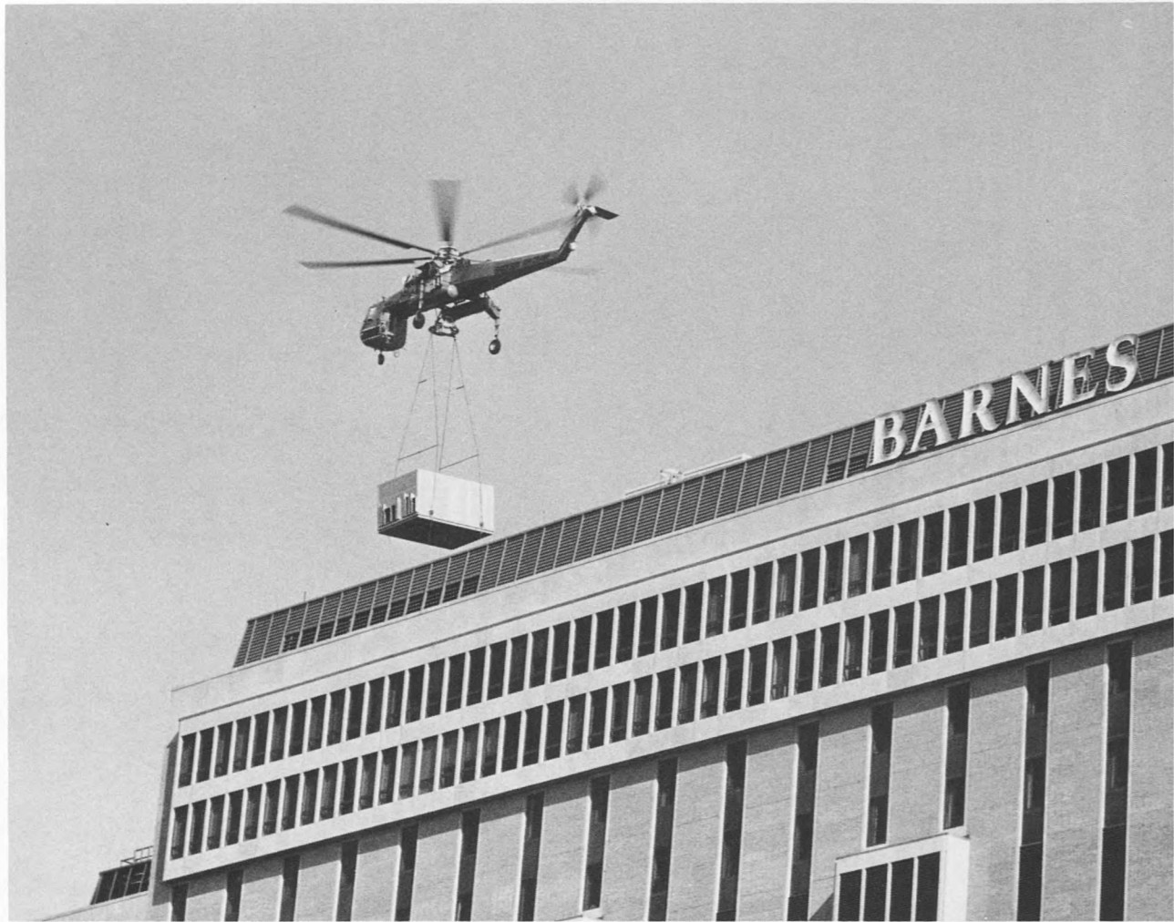
A large, orange "Skycrane" helicopter hovers over Barnes Hospital with a cargo of new air conditioning equipment en route to Queeny Tower rooftop. Each of the three units transported September 13 weighed approximately 15,000 pounds and was moved in two to three sections. The four-hour maneuver between a storage lot at Clayton and Boyle avenues and Queeny Tower necessitated the temporary closing of streets in the flight path to non-emergency vehicles.
