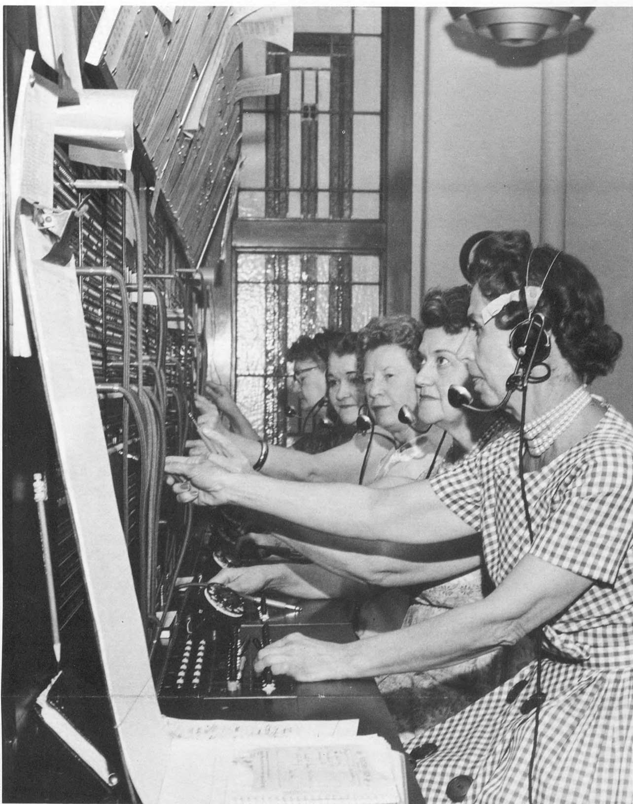
In 1962, operators manned a 1,000-station switchboard and handled a daily task load of 20,000 routine and emergency calls. Barnes boasted of having the largest hospital communications system in St. Louis.
