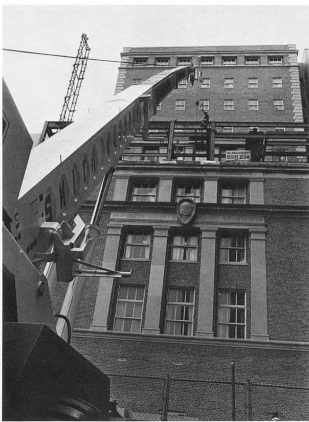
Construction is progressing rapidly on Mallinckrodt's new NMR facilities.
