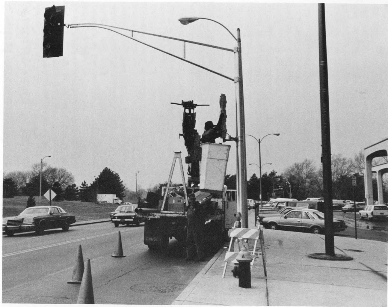
Traffic signals were recently installed on Barnes Hospital Plaza at the entrance to the subsurface garage. The signals were installed for the protection of visitors and employees crossing the street, as well as to aid those persons trying to drive out of the garage onto Barnes Hospital Plaza.
