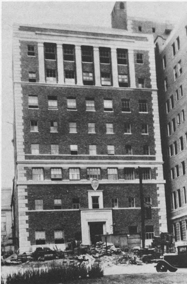
MIR's original building as it was nearing completion in 1931. It faced Kingshighway and abutted Barnes' Rand-Johnson building. Later additions added four floors atop the building and five floors in front of the original entrance.
