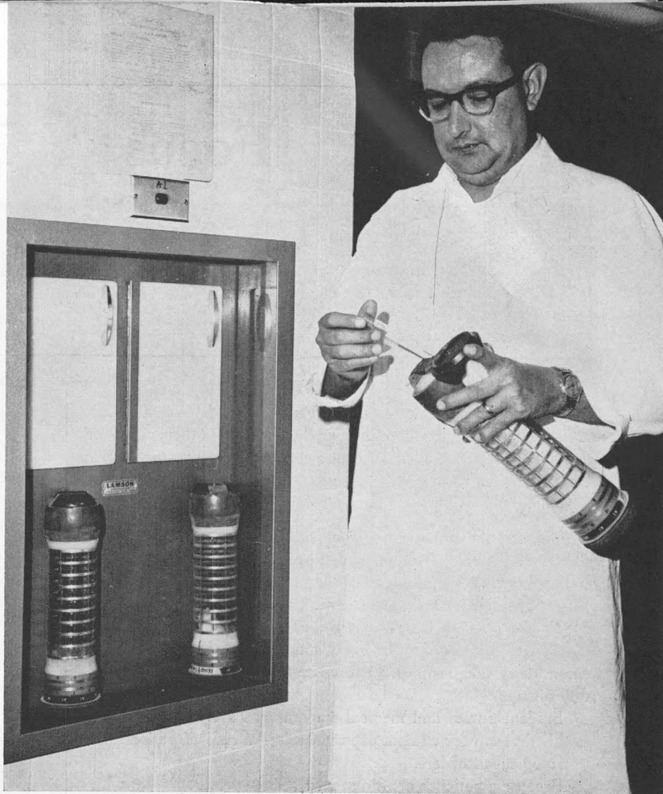
THE PNEUMATIC TUBE SYSTEM is used frequently by the diagnostic lab. Here, N. Gonzales-Rubio, head technician, removes a blood sample which will be analyzed in the lab.
