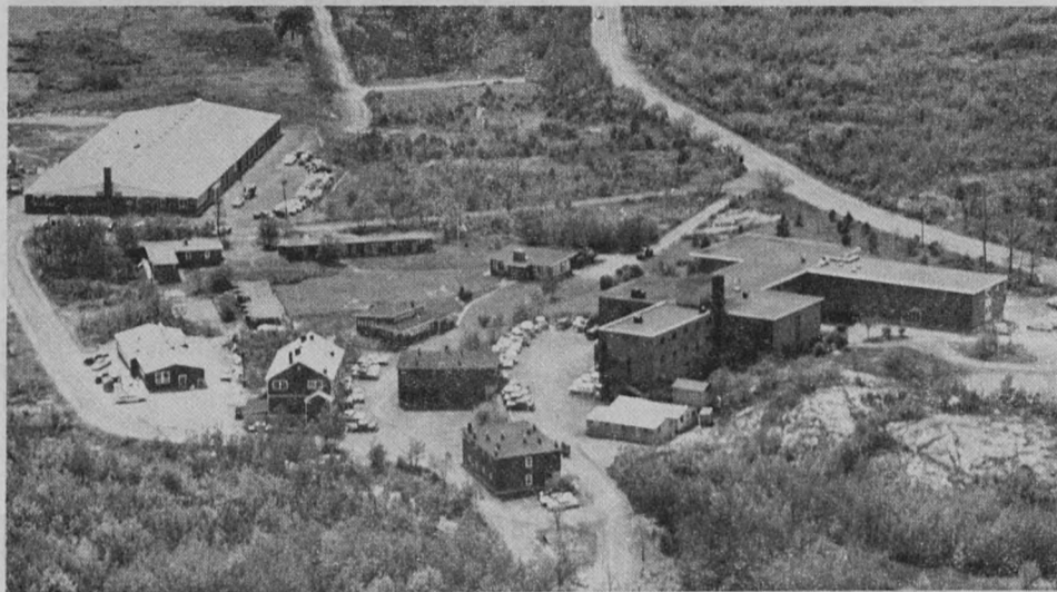
AERIAL VIEW of the Main Laboratory complex of the Roscoe B. Jackson Memorial Laboratory. Upper left: Morrell Park Laboratory. Lower left: Animal Health Research Laboratory. At right is the Main Laboratory, which houses a large part of the Laboratory's research program.
