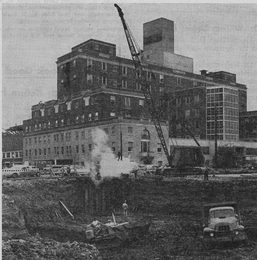
Tunnel construction: A new view of Jewish Hospital (see story, left).
