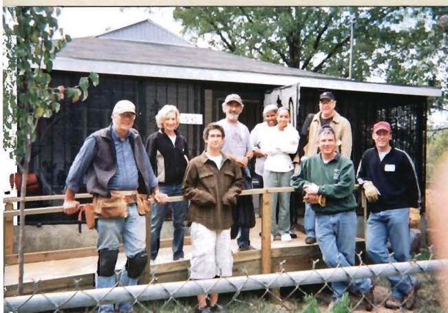
Dallas – Washington University volunteers and a delighted homeowner show off a completed home access ramp. The Dallas Ramp Project builds about 200 ramps per year for area residents.
