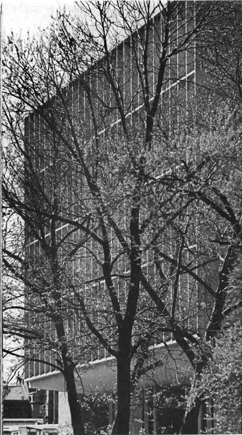
Nature does her bit also by clothing the trees in bright green buds and accenting the soaring lines of a new building.
