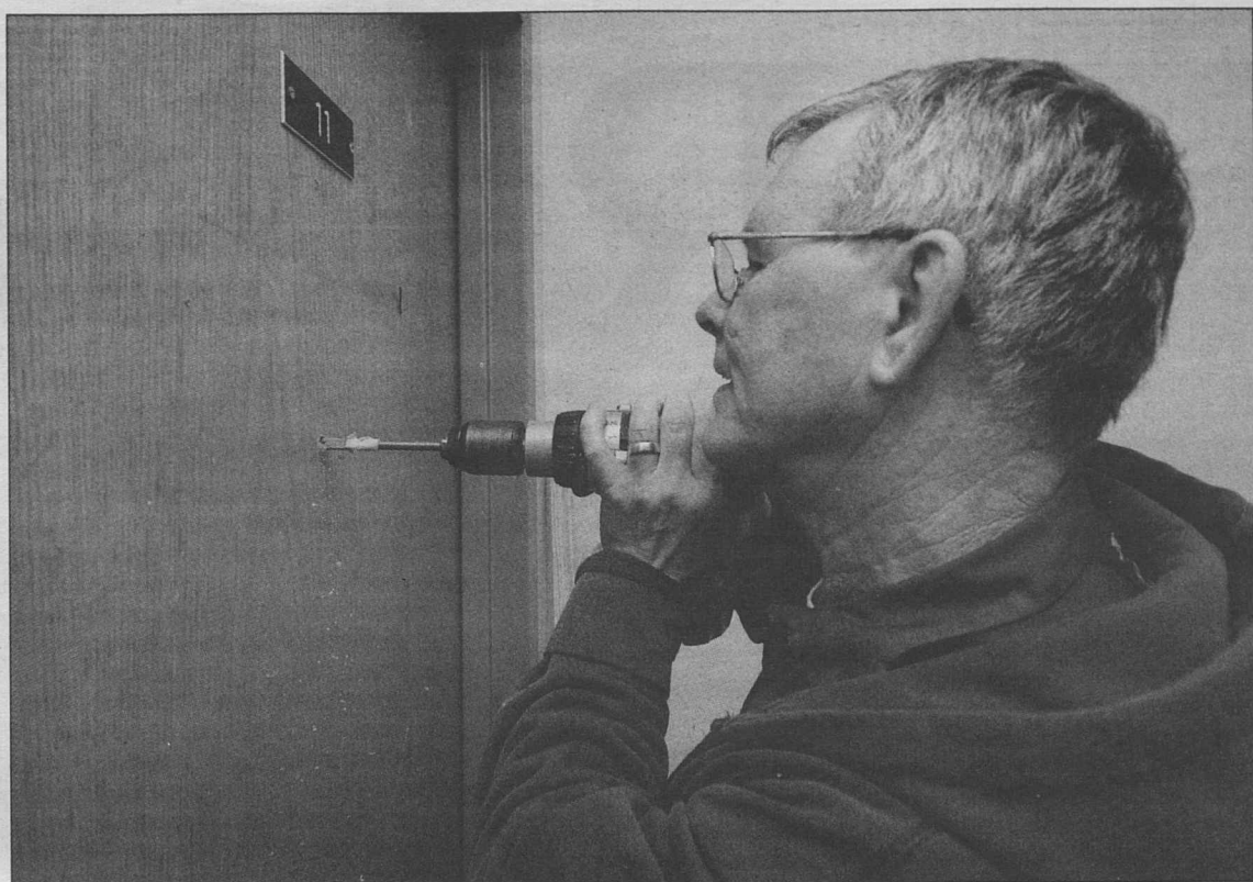
Tom Biehl, a mechanic with Maintenance Operations, installs a peephole in the door of a Hurd House dorm room. Seven two-man crews installed peepholes in residence hall doors last week as an added security measure for students.
