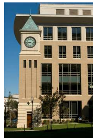
View of the Clock Tower and Wolff library
