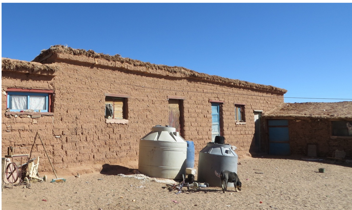
Figure 8. House built of adobe with roof made of straw located in Casa Colorada (40 km from San Antonio de los Cobres). Tanks contain drinking water. Photographer: Florencia Harari.
