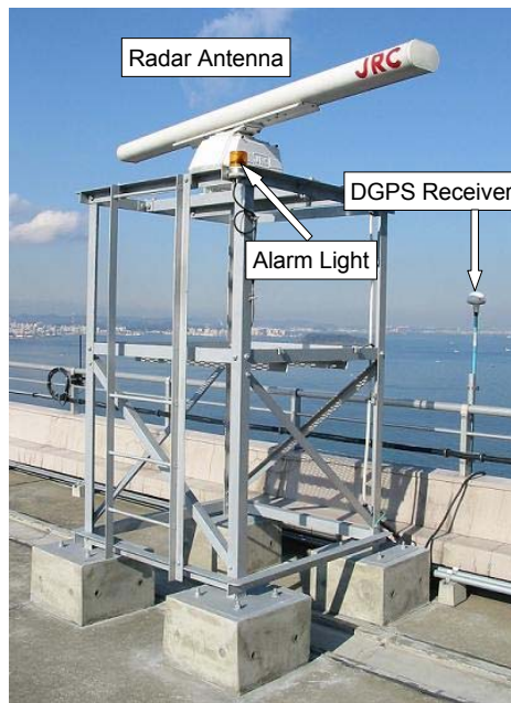
Fig. 2.4 Radar structure
